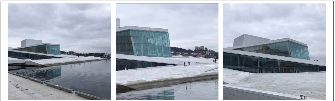
The Oslo Opera House
