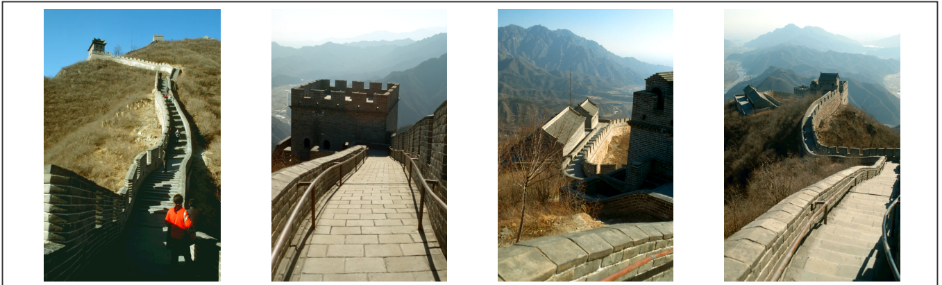
The renovated section
