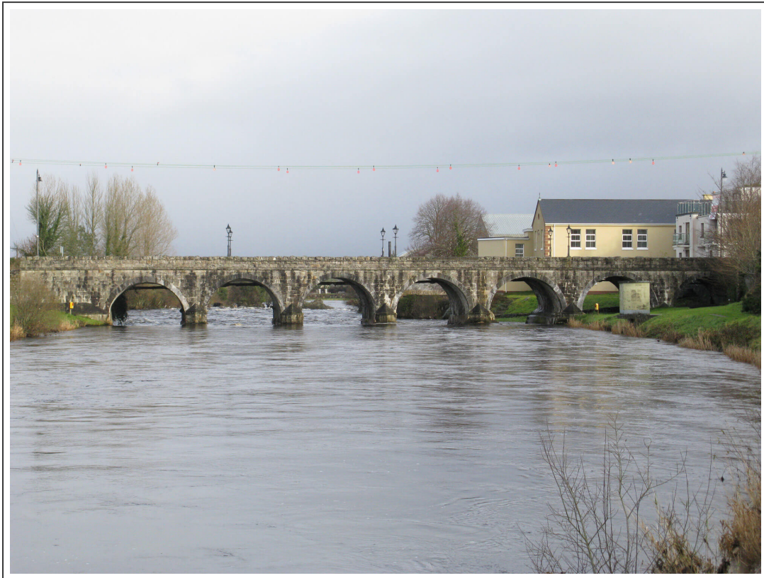
The bridge over the May river in Foxford
